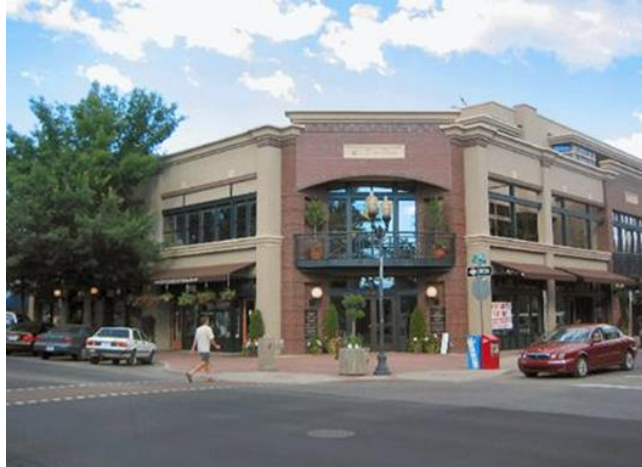
Corner lot development featuring the primary entrance oriented toward the corner.
